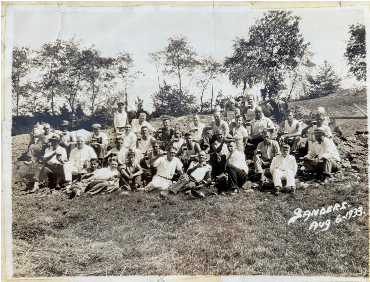
Post Members digging foundation for the Post 210 Building on North Street Doylestown.
